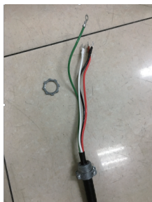
Remove the ring by turning counterclockwise
